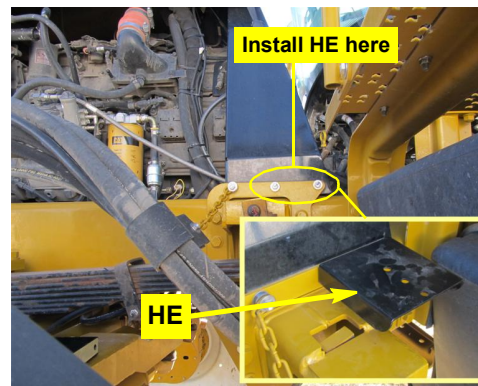
Figure 2 with inset: Installed steering block mounting bracket
