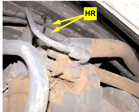
Figure 5c-iii: Steering hoses routed to steering block
