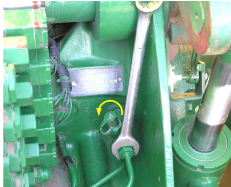
Figure 2: Retightening test port fittings (port rotated)
