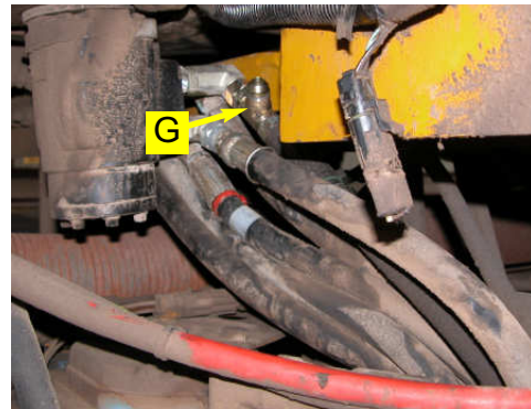
Figure 3b. Run tee installed.
