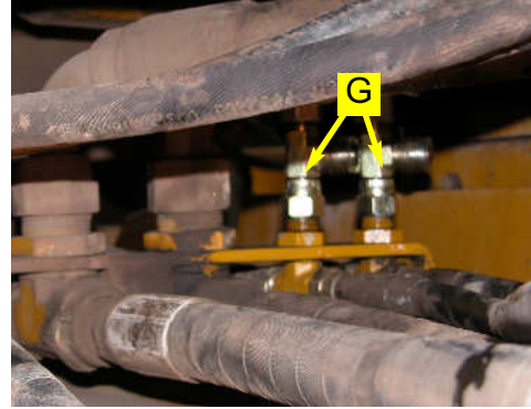
Figure 5b. Installed run tees.
