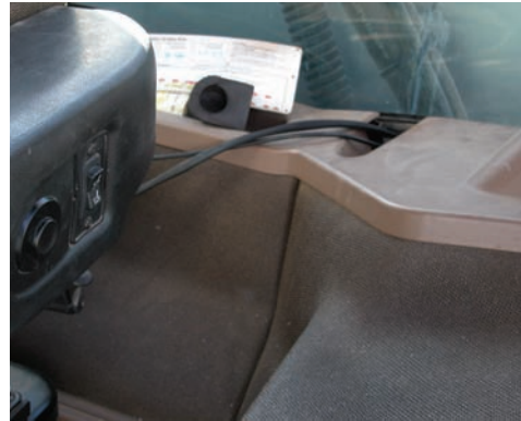
Figure 8b: Cab access hole
