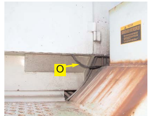
Figure 7b. Valve cable routed in cab.
