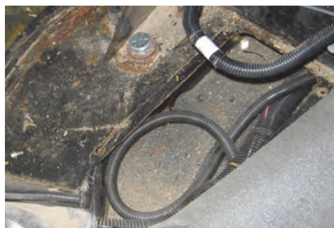
Figure 1: Example pre-drilling check
