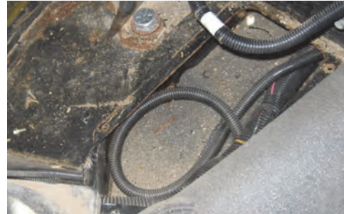
Figure 1: Example pre-drilling check
