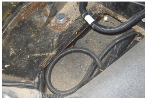
Figure 1: Example pre-drilling check
