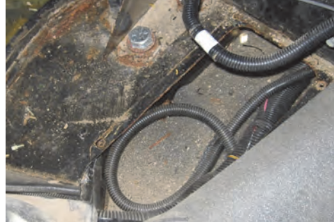
Figure 1: Example pre-drilling check
