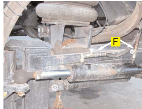
Figure 5b. Installed run tees.
