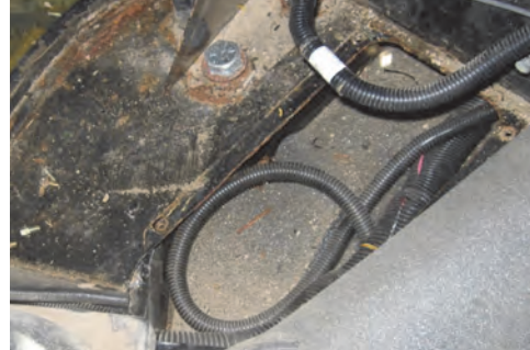
Figure 1: Example pre-drilling check
