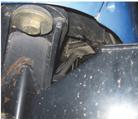
Figure 2c-i: PVE and WAS cables routed through the cab access hole
