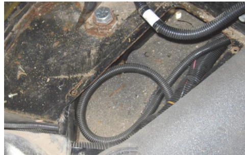
Figure 1: Example pre-drilling check
